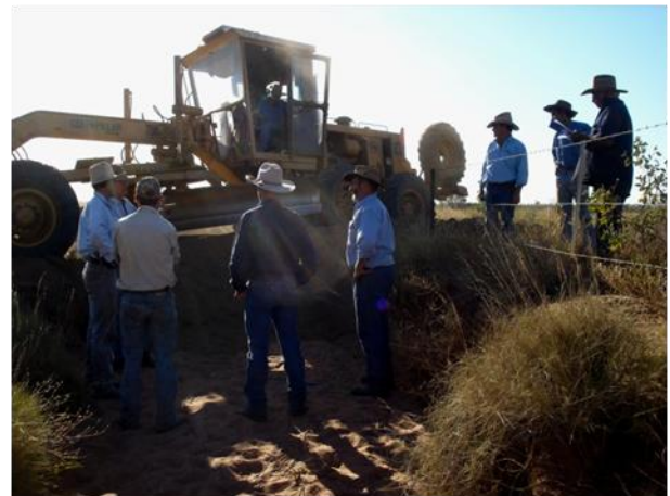
Constructing a diversion bank at Jubilee Downs
