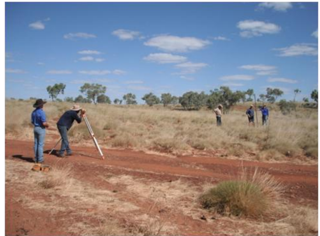
Pegging out a diversion bank at Larrowa Station
