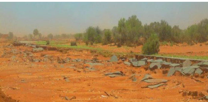
What remains of a section of the road to Gascoyne Junction. First flood, then dust storm, and followed by locusts.
